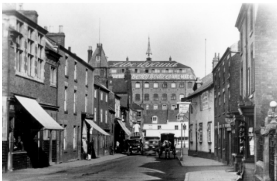
THE BELL INN, COVENTRY ROAD, MARKET HARBOROUGH. (WHITE BUILDING ON THE RIGHT).
