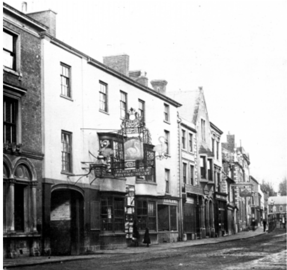
THE THREE SWANS HOTEL IN COACHING DAYS. FURTHER ALONG THE HIGH STREET IS THE COACH AND HORSES INN DEMOLISHED IN 1901 ALONG WITH ROWS BUILT IN ITS YARD AND WATERFIELD PLACE TO MAKE SPACE FOR ABBEY STREET.
