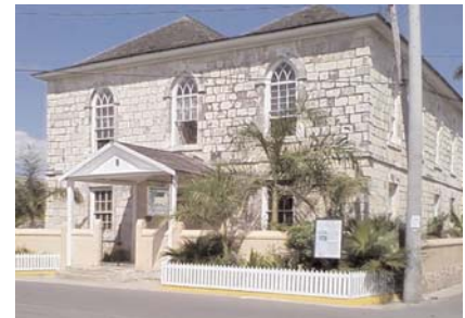
Now known as the Baptist Manse, the building on the corner of Market and Trelawny Streets, Falmouth, was built as a Masonic Temple in 1798.
