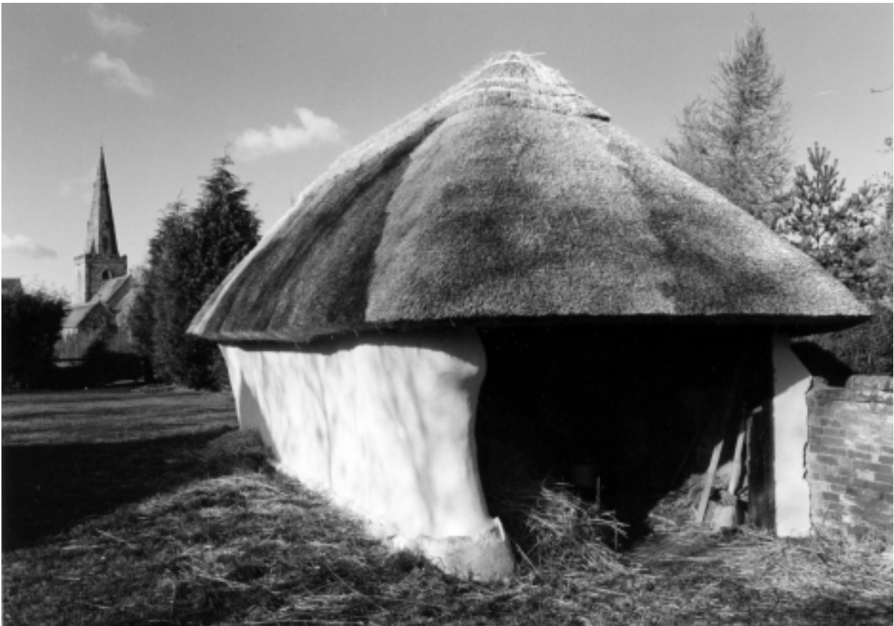
HOVEL AT GILMORTON RESTORED IN 1996.
