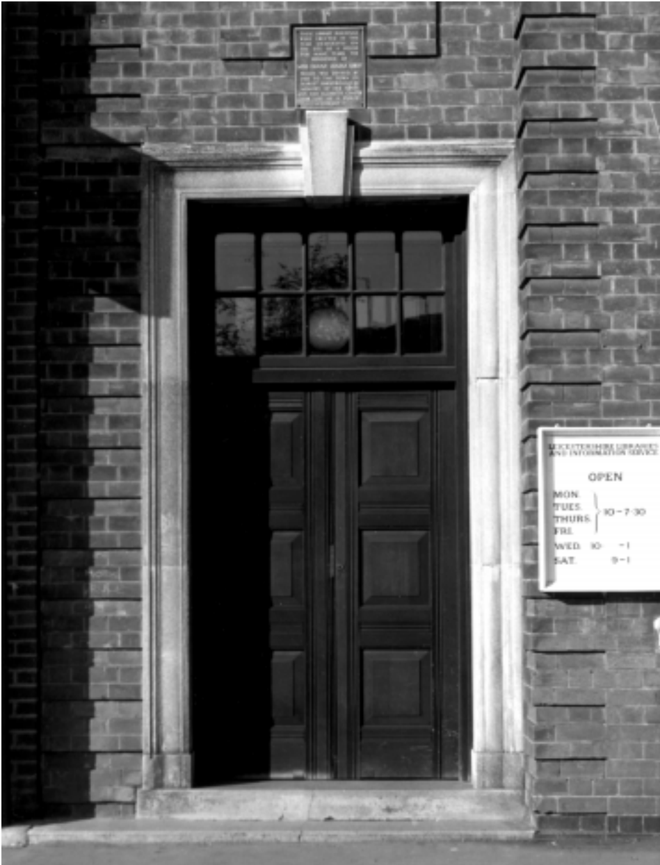
DOOR OF FORMER LIBRARY 53 THE SQUARE, MARKET HARBOROUGH 1981.
