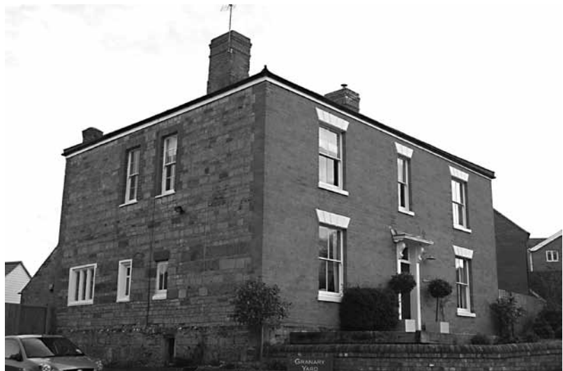
FARRER FARM IN EAST FARNDON. SOME OF THE STONE WORK IN THE SIDE WALL IS LIKELY TO BE PART OF THE ORIGINAL (18TH CENTUR?) BUILDING, THE REST BEING PART OF H.M. VANE'S 1865 ENLARGEMENT.
