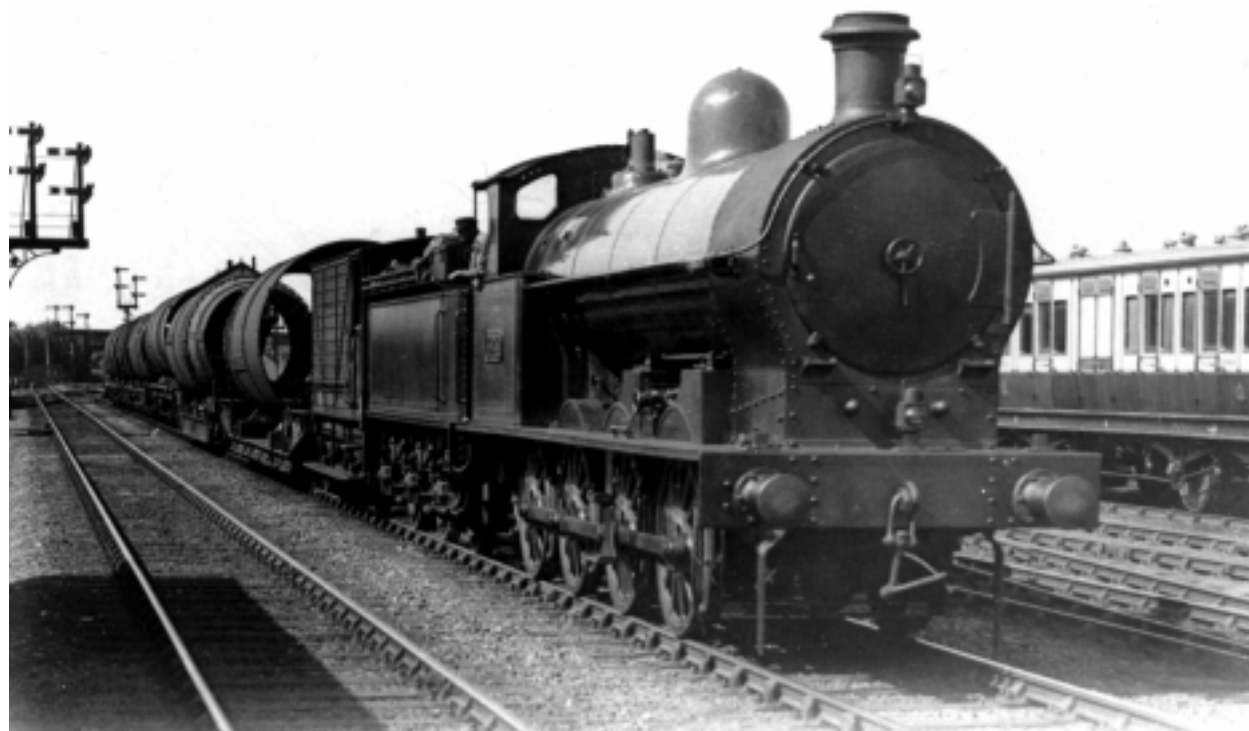
PARTS OF KILNS BEING MOVED FROM BARROW-IN-FURNESS TO POPLAR, NORTHAMPTON MAY 1921.
