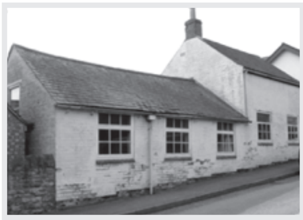
These outbuildings on Farndon's Main Street were once used as a laundry. The 1901 census records four women as laundresses and it is most likely that they worked here.
